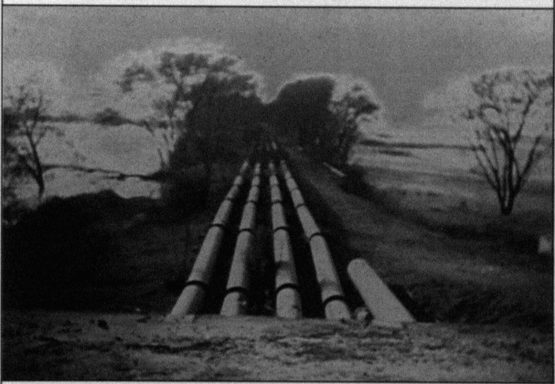
Hume pipes carrying ash from thermal plant to ash tanks within Wetland
